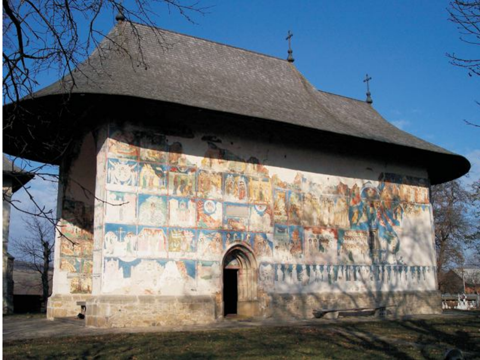
Fig. 1 - Arbore, South façade.
